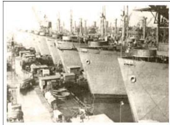
The design was modified by the USA Maritime Commission to conform to American construction practice and to make it even quicker and cheaper to build. The USA version was designed "EC2-S-C1" for emergency cargo. The new design replaced much riveting, which accounted for one third the one third of the labor costs with welding and featured oil fired boilers.
